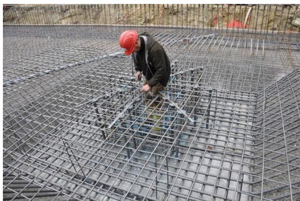
Armatures anti-poinçonnement de la dalle parking
